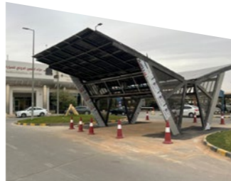
Solar-powered canopies were installed in the auction center's parking lots.
